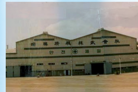
→ Constructed casting plant in Pohang
