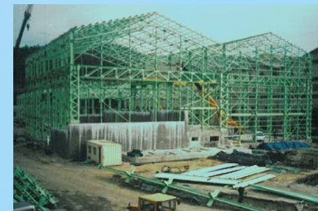
→ Construction site of the 2nd casting plant in Pohang
