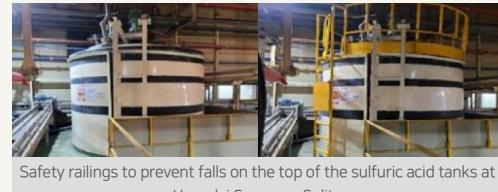
Safety railings to prevent falls on the top of the sulfuric acid tanks at Hyundai Sungwoo Solite
