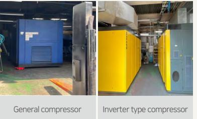
1 Excessive power usage due to aging compressor equipment and insufficient air supply has been addressed by installing three inverter-type compressors.
