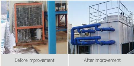
Excessive power consumption caused by cooling the rectifier rooms with chilled water from the refrigeration unit has been improved as follows.
