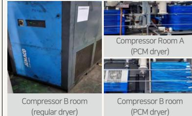
Power consumption issues caused by using conventional refrigerated dryers have been improved by installing PCM (Phase Change Material) dryers.
